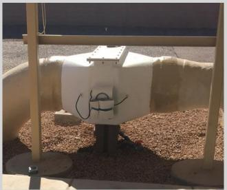
FanAir Co. 3000 CFM, 2 Stage Mist Eliminator and Mesh Pad moisture separator used to eliminate moisture on inlet side of centrifugal blower for a Carbon Absorber.
